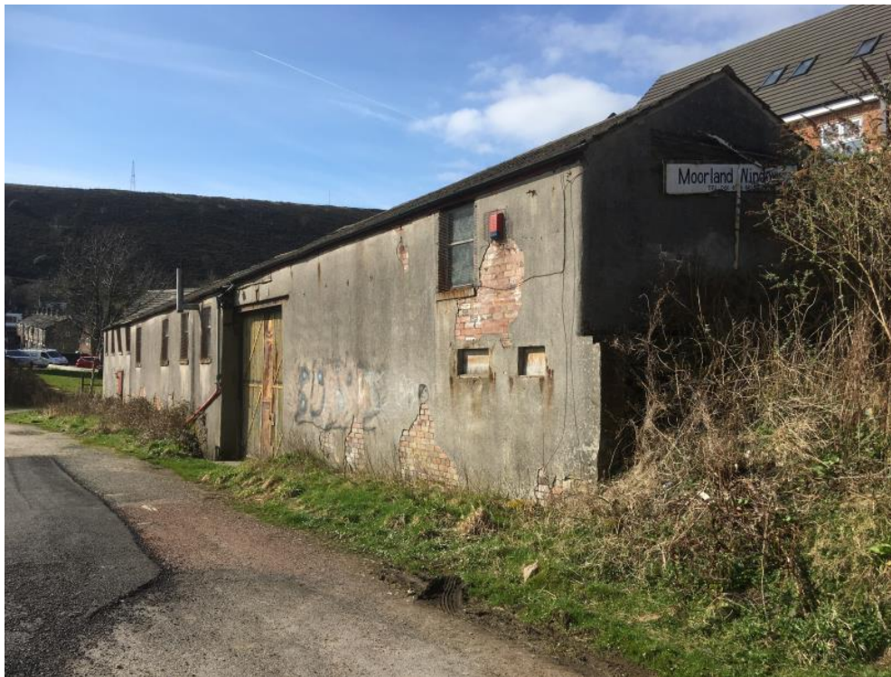
Photo 4: Warehouse to be demolished
