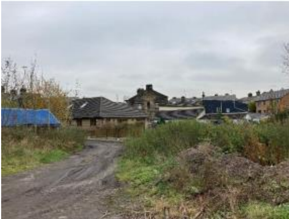
Photo 7: Retaining structure on the northern boundary to Shire Croft properties.
