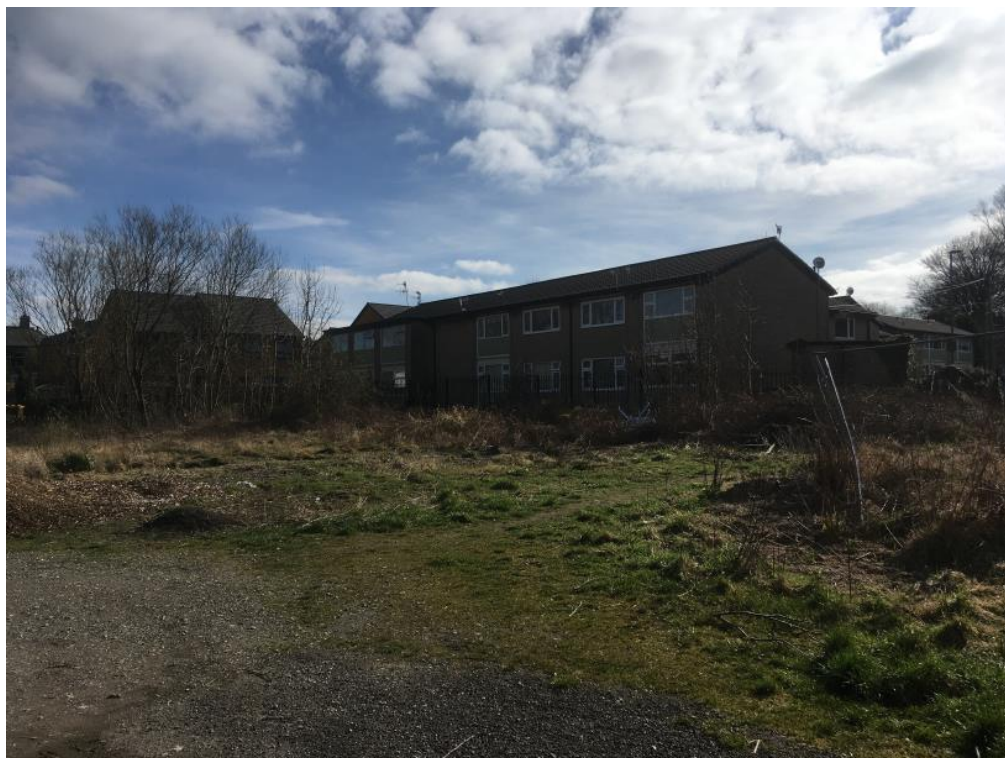
Photo 5: View to the South Western boundary
