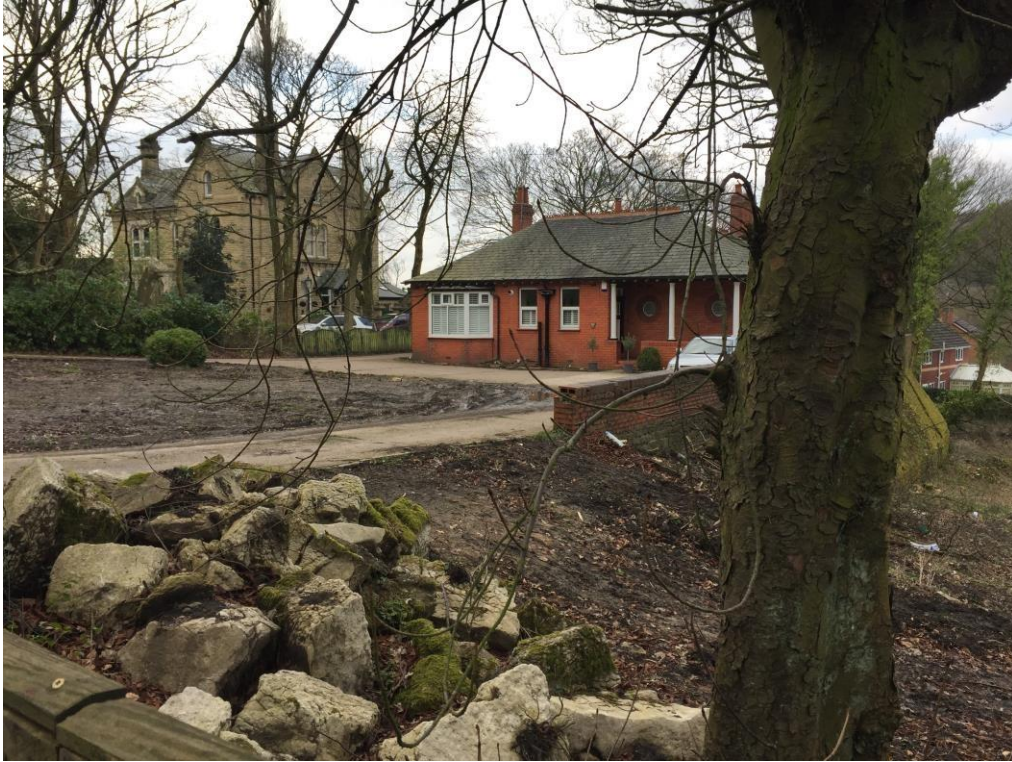
Photo 1 – view of Existing property at 164 Mottram Road and neighbouring property to the south
